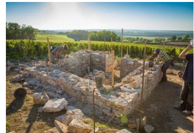
Fig. 67. Base of a vineyard hut, France. Built by Laviors et Murailleurs de Bourgogne (Burgundy Stone Roofers and Wallers). Photo: Johan Mari.
